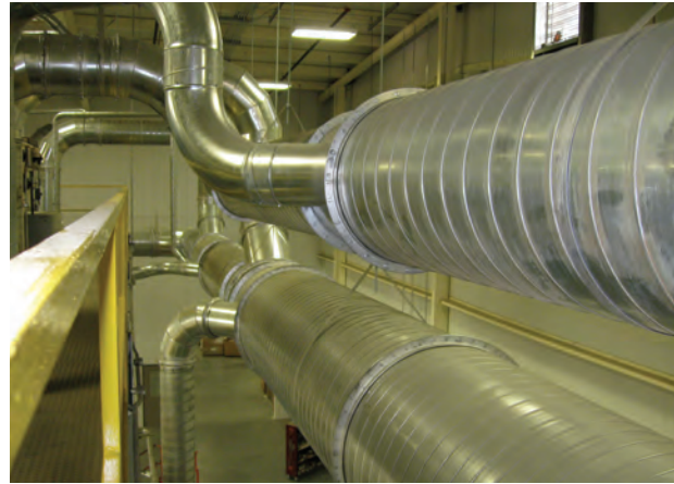
Spiral pipe can ship with flanges for easy installation.
