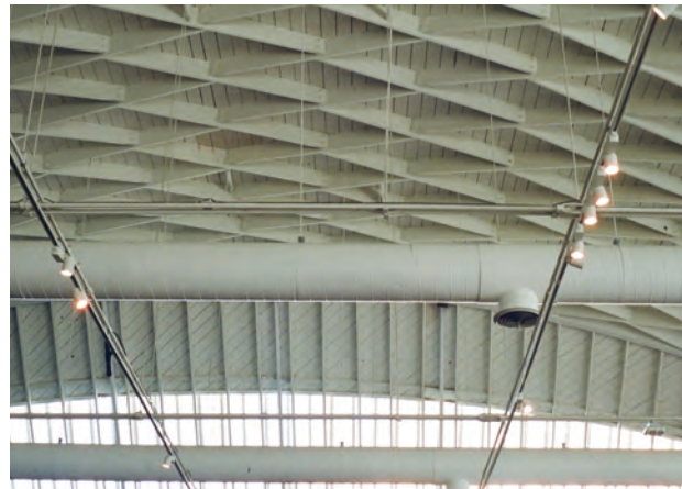
Spiral pipe in galvanized steel (paint grip material).
