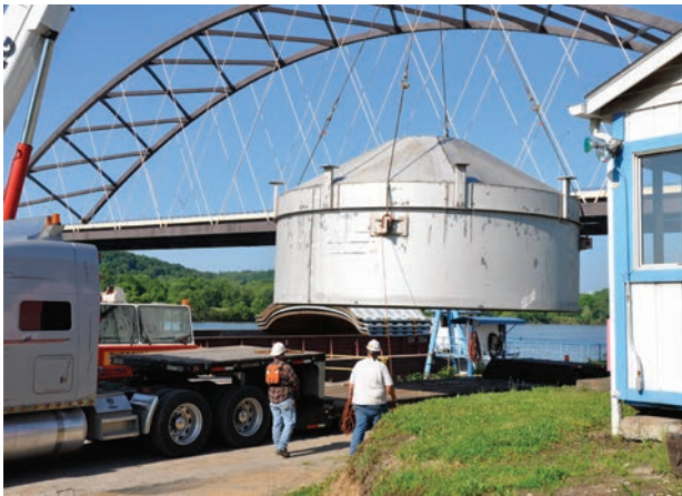
Loading Danser-fabricated 22' diameter Alloy 800H vessel top section onto barge for shipment.
