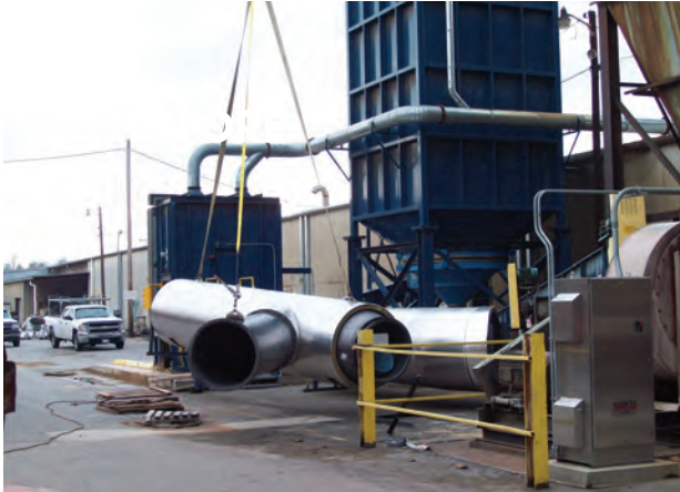
Installing new exhaust duct section during plant shutdown.
