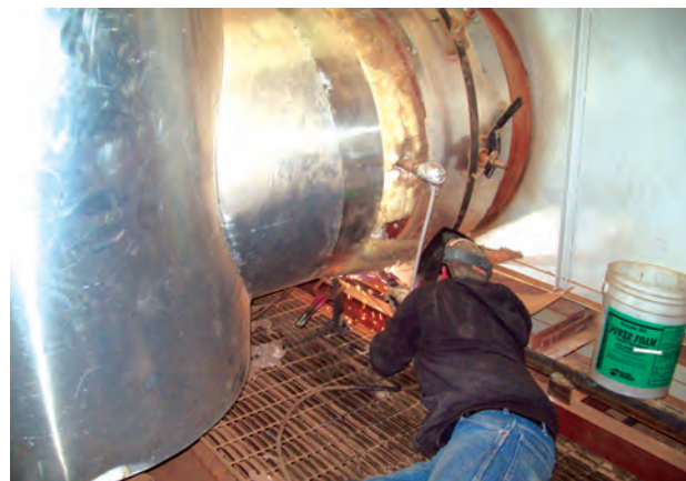
Danser crew repairing damper.
