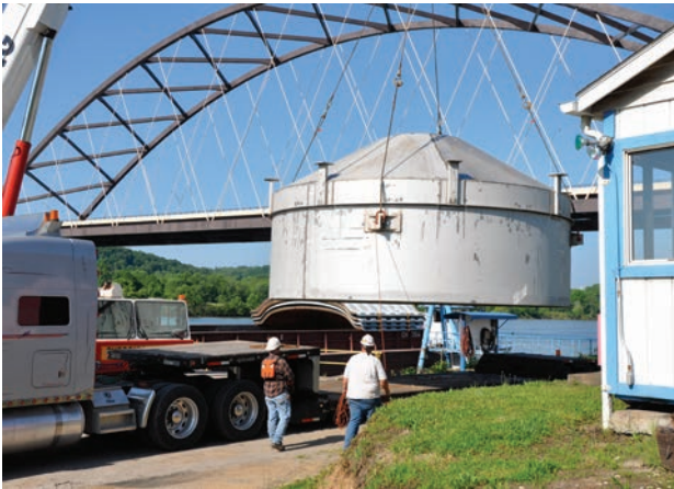
Loading Danser-fabricated 22' diameter Alloy 800H vessel top section onto barge for shipment.
