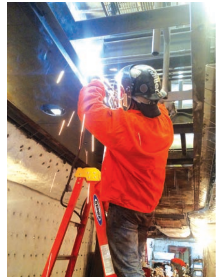
Danser crew repairing furnace during customer holiday shutdown.
