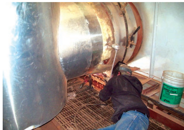
Danser crew repairing damper.
