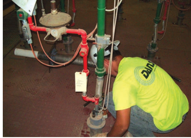
Changing gas burner while the kiln is still running, avoiding expensive downtime for the customer.
