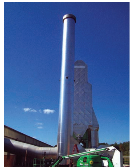
New insulation & lagging installed on customer's exhaust stack, as well as baghouse upgrades during planned shutdown.
