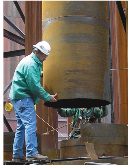
Danser fabricated and installed cooling U-Tubes at specialty metals plant.
