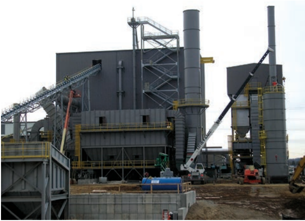
Danser fabricated & installed pollution control equipment, ductwork, structural steel, conveyor, exhaust stack.
