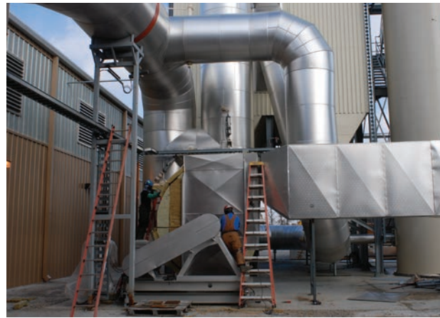
Installing Danser-fabricated ductwork, insulation and lagging.
