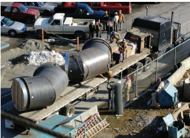
Danser crew prepares to install ASME B31.3 process pipe for a steam reformer. Pipe fabricated by Danser.
