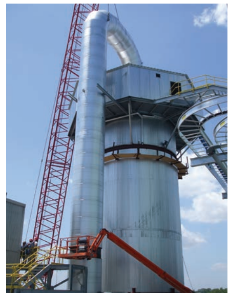
Installing Danser-fabricated inlet duct on 80' tall spray dryer (also built and installed by Danser).
