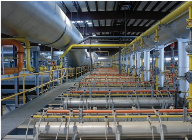
Danser fabricated & installed combustion piping, air headers, fresh air & exhaust duct with insulation & lagging.
