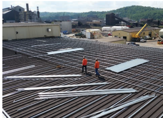
Danser crew retrofitting metal roof with Hat Channel, Z-Bars and 75' long sheets.
