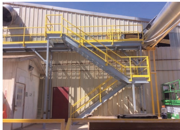
Danser detailed, fabricated and installed access stairs and platform.
